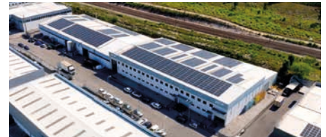
OIÁ PLANT • Covered factory area: +10.000 m 2
